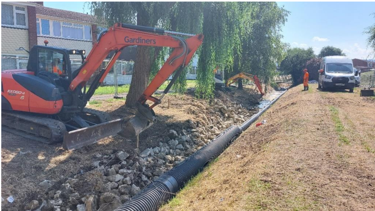
During works - removal of concrete channel
