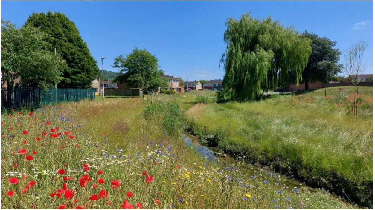
Completed works – natural, sinuous, 2-stage channel, with riparian wildflower meadow
